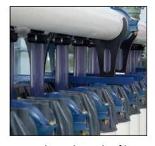
mg/l suspended solids is possible). The larger diameter reduces the pressure drop along the fiber significantly in comparison to smaller capillaries. This results in a more even water distribution along the fiber and consequentially in a more evenly distributed fouling layer. Thus, the removal of the debris by backwashes is more efficient and usually results in savings on necessary membrane area.
